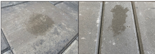
Surfaces ready to be sealed
